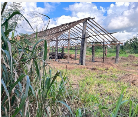
The structure of the 2nd hut is in place.
